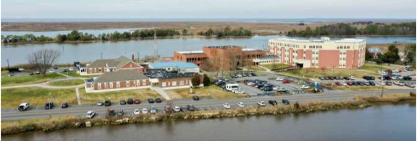
Figure 6-4: Image of Tidal Health – McCready Pavilion. Source: https://www.tidalhealth.org/our-locations/tidalhealth-mccready-pavilion
